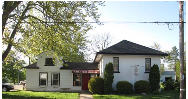
Existing Maple Acre Library in Fenwick
