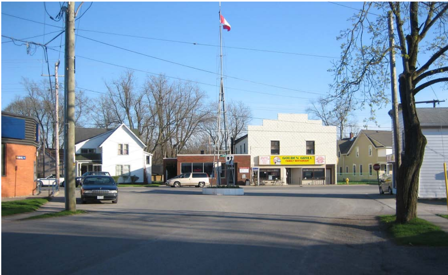
Before | View looking south on Maple Avenue, towards Canboro Road. At present, the view terminus is the flagpole, post office, and Golden Grills Family Restaurant. A single-storey commercial building currently occupies the north-east corner at the intersection (left).
