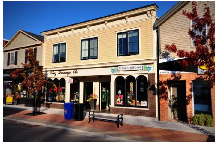
Recently renovated buildings with façade improvements in Fonthill.
