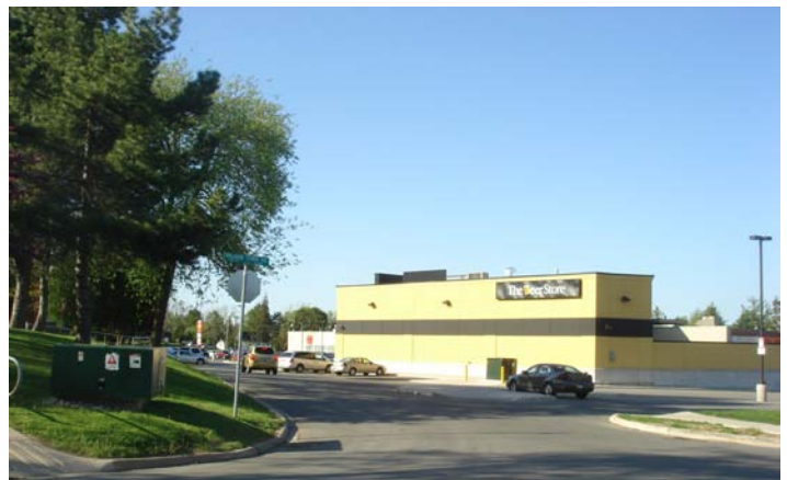
Current built form conditions along Pelham Town Square: One- to two-storey buildings set back far from the street, proliferation of front driveways and parking areas visible from the street
