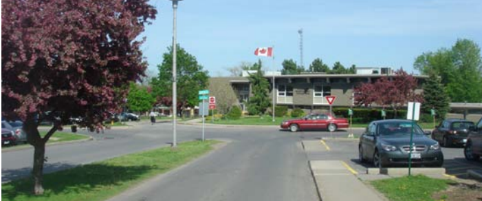
Existing Town Hall in Fonthill
