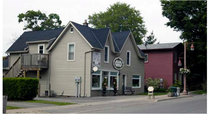
Preserved historic buildings in Ridgeville, Canboro Road
