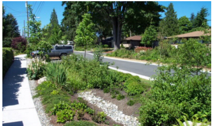
Example of vegetative or grassy swale drain
