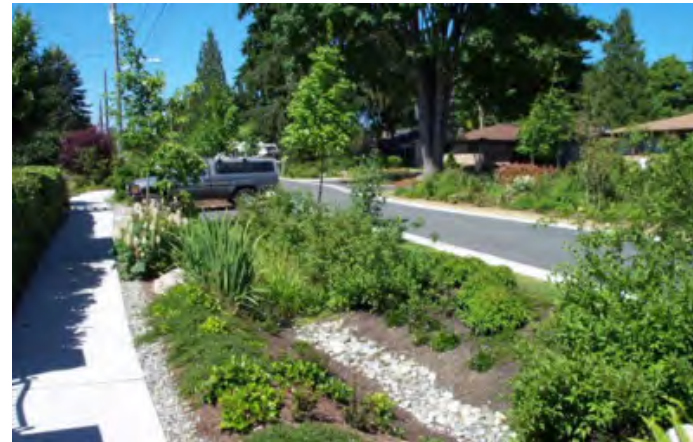
Example of vegetative or grassy swale drain
