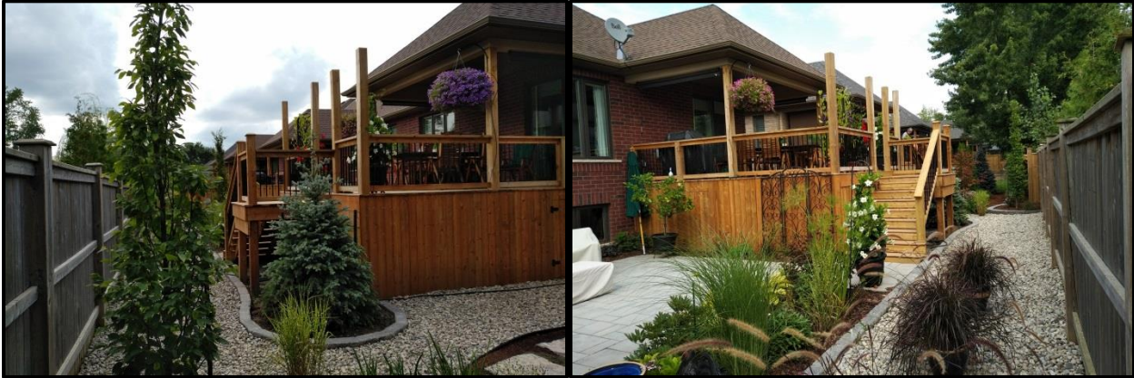
Figure 2: Unfinished deck extension at 12 Brayden Way
