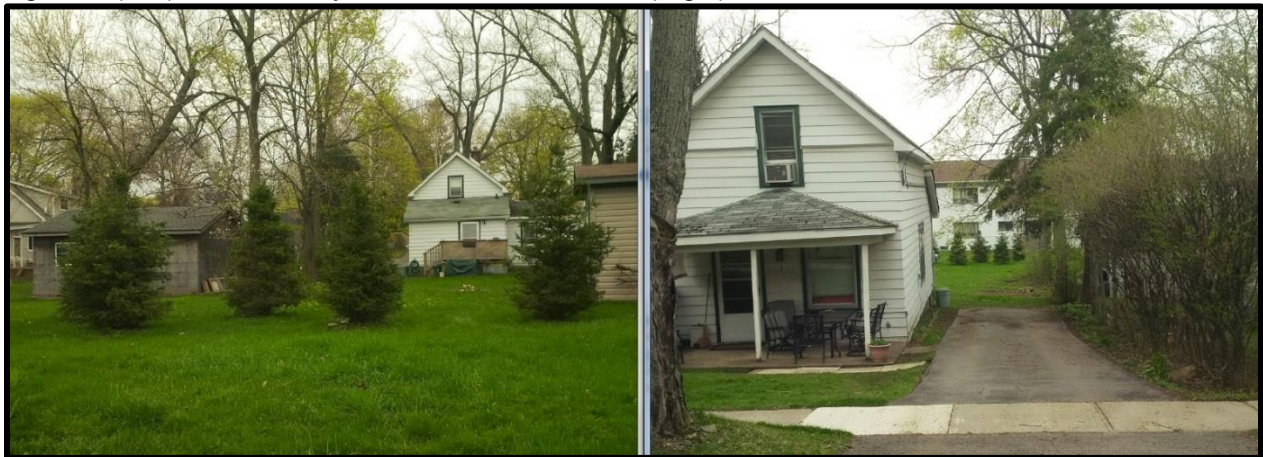
Figure 1: (Left) View of rear yard from Short Hills land, (Right) View from Linden Ave
