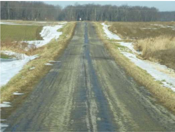
Figure 11. Balfour Street, from River Road to Webber Road (RR29) – LCB
