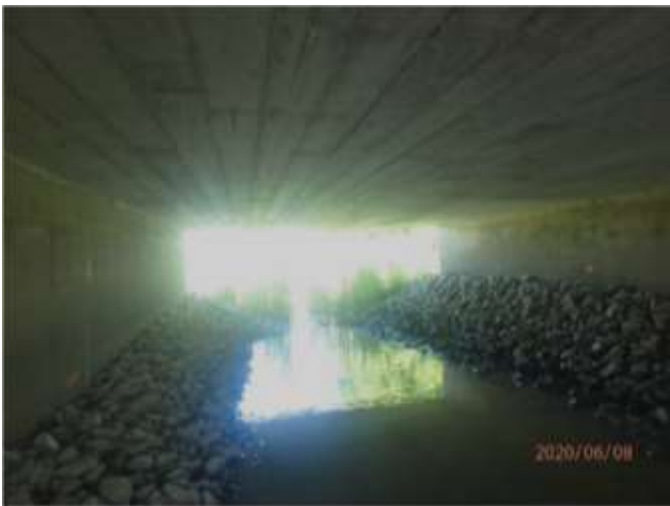
Figure 17. Interior looking east.
