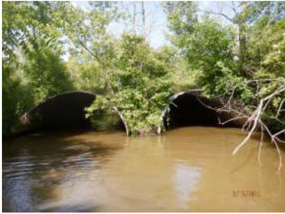
Figure 23. East end of pipes.
