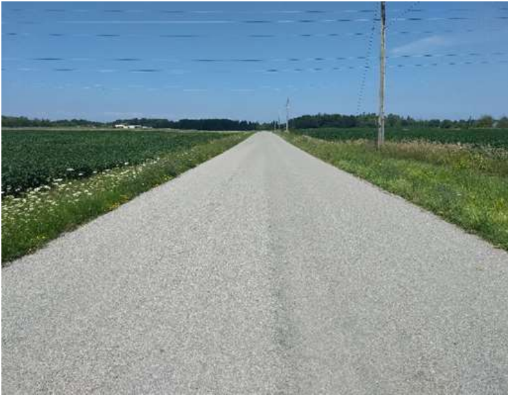
Figure 8. Maple Street, from Sixteen Road to Roland Road – LCB
