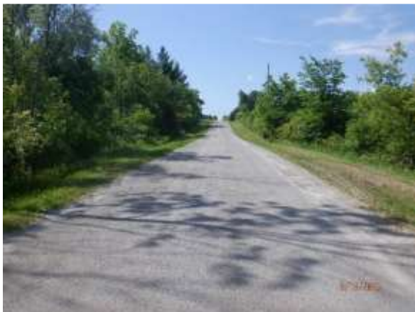
Figure 22. Roadway over structure looking south.
