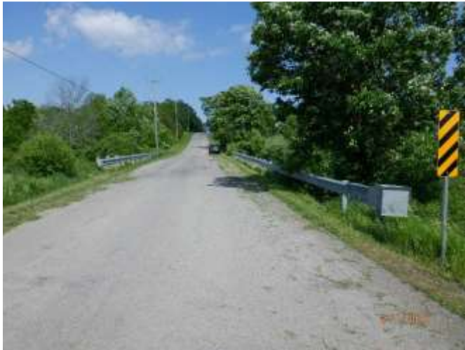
Figure 18. Roadway looking east.
