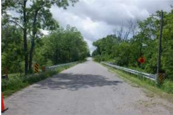
Figure 26. Roadway looking west.
