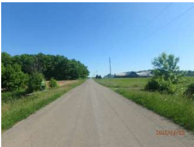
Figure 14. Surface treated roadway looking south.
