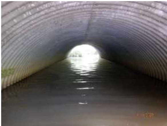
Figure 24. Interior of south cell, looking west.
