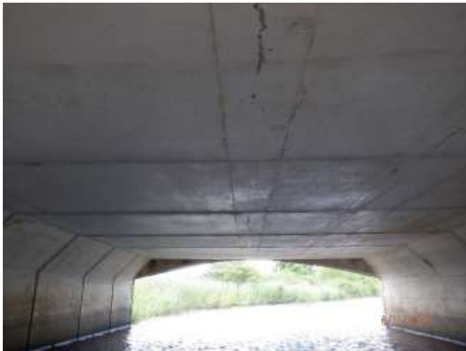
Figure 19. Interior of structure, looking north.
