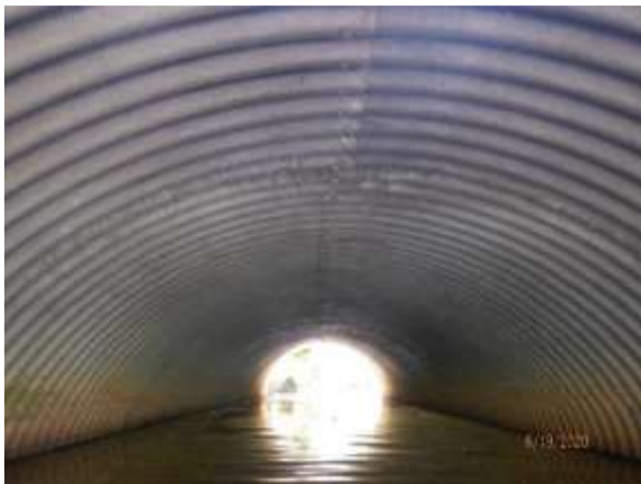
Figure 25. Interior of north cell, looking east.
